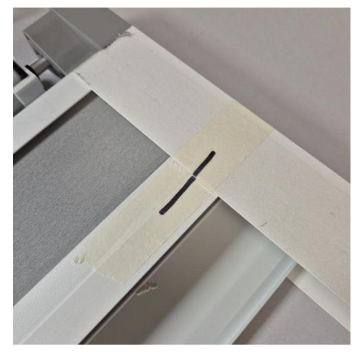
Ensure that the black lines on the float rail align with the black lines on the side channels.
