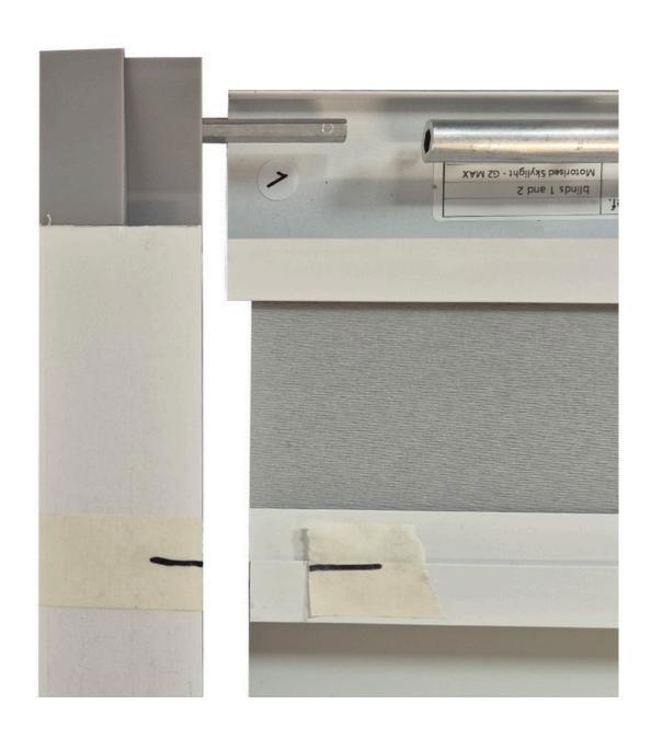
Rest the side channels of each blind onto the shelf (main gearbox end), and push the sub-gearbox ends into the join covers.
